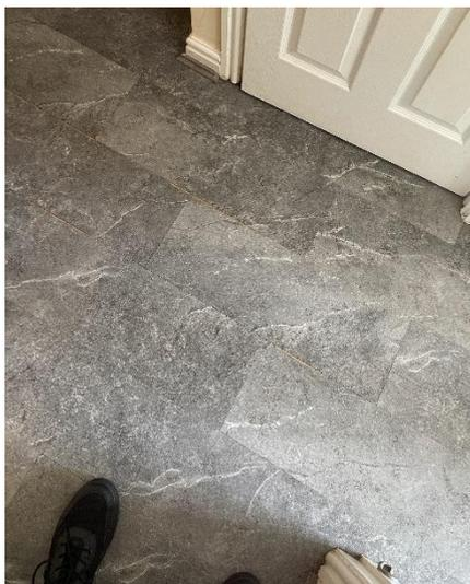
This floor had a lot of movement underfoot when walked over, which was caused by an uneven subfloor and use of additional (laminated) underlay. After a period of just 5 months, the floor had broken on many joints due to stress on the joints of the click system.
