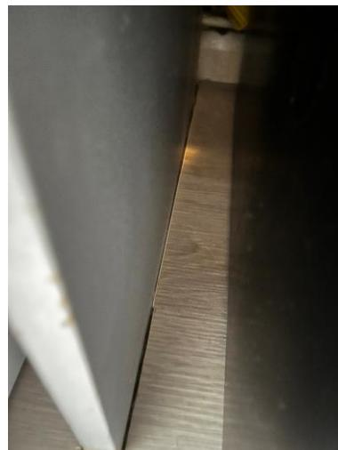
Even cuts around kitchen units require adequate expansion gaps as the floor can expand in multiple directions when the temperature changes.
